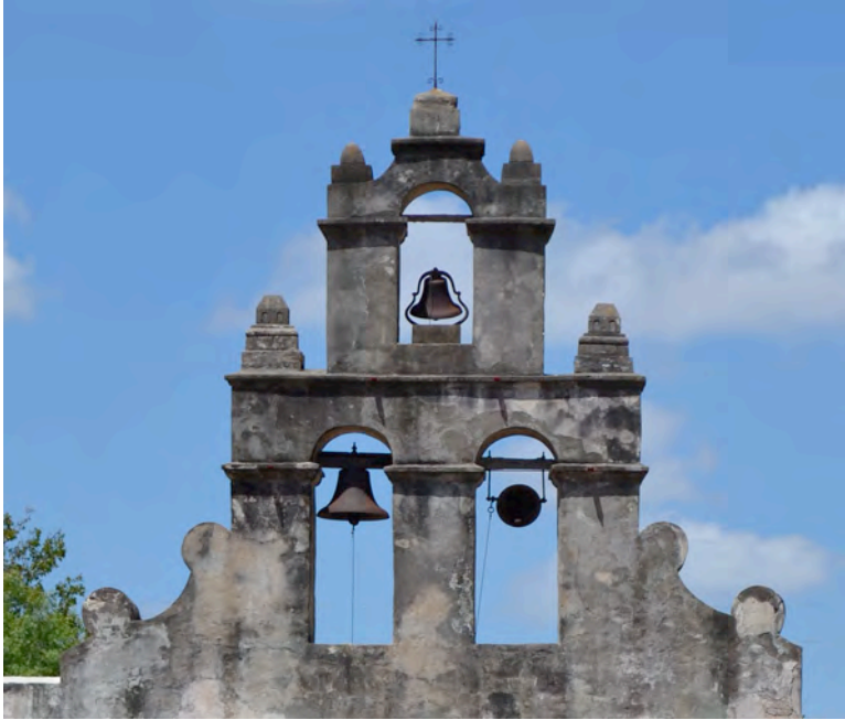
Plate 5. The bell tower is comprised of two tiers of masonry arches now covered with stucco. Photograph by author.
