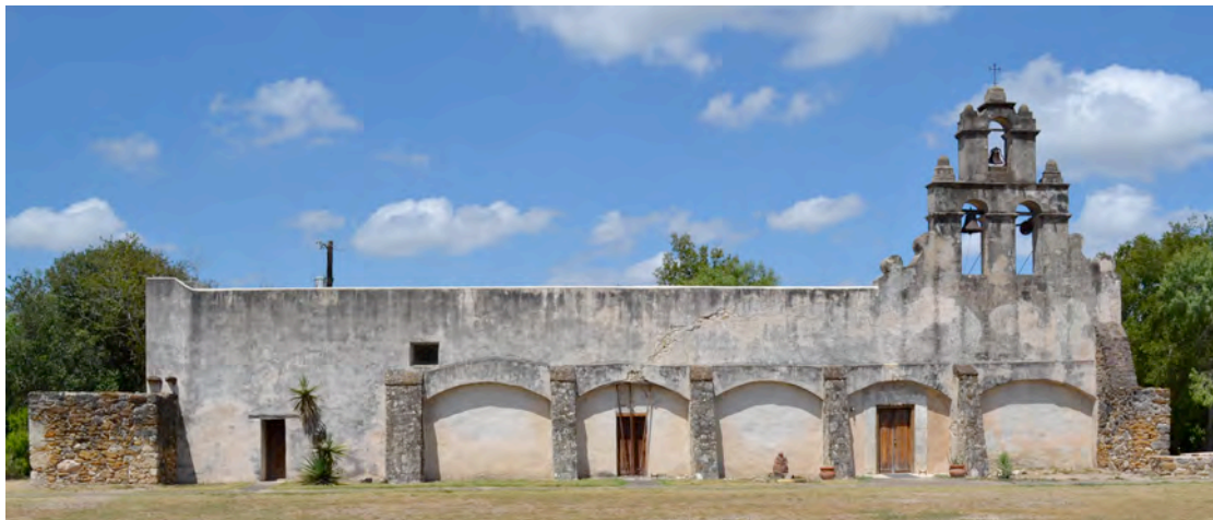
Plate 2. The east elevation of the chapel with adjacent boundary wall remnants to north and south, as viewed from the center of the Mission plaza. Photograph by author.
