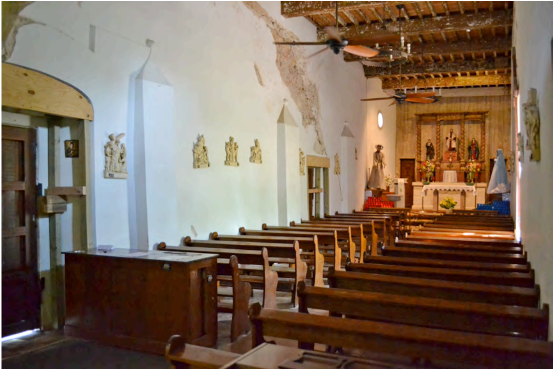
Plate 6. View from the back of the nave looking south toward the altar, as it appeared immediately prior to renovation in August 2011. Photograph by author.
