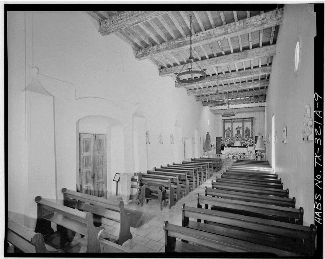
Plate 7. Interior of church and altar in 1983. Photo by Jet Lowe. Courtesy Library of Congress. Prints and Photographs Division. HABS TX-321 A-9.
