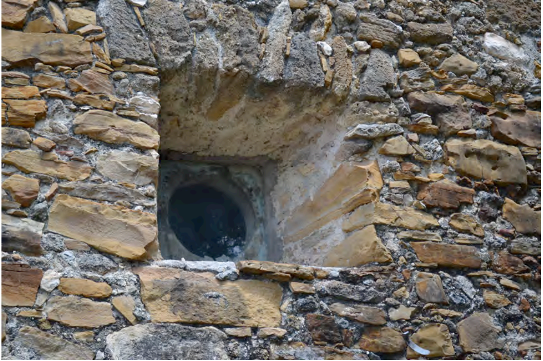
Plate 9. Ocular window at northwest corner of nave. Photograph by author.
